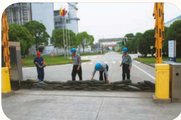
Piling Sandbags for Flood Prevention
