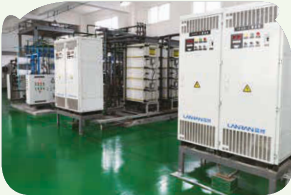
Desulfurization Wastewater Treatment Facility
