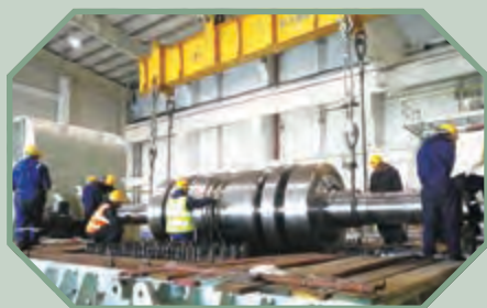
Retrofitting construction site of the low-pressure cylinder light- changing shaft of No.1 unit steam turbine
