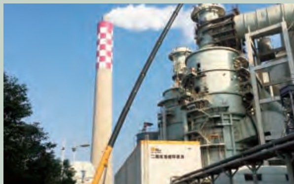
Hoisting operation of absorption tower retrofitting
