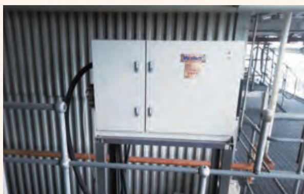
During unit maintenance period, CR Power Bohai New Area Power Plant installed a WalsnCEA-828 fuel efficiency analyser in front of each flue AIG of No.1 boiler so as to ensure the economic feature of burning by maintaining appropriate CO content, thus reducing its net generation standard coal consumption rate by approximately 0.30 g/kWh and saving approximately RMB 767,100 a year.
