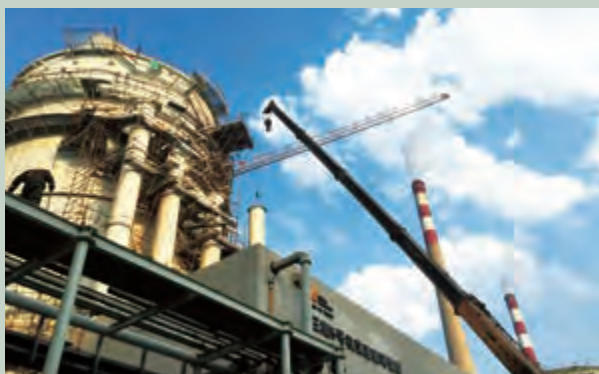
Ultra-low emission retrofitting site (hoisting operation of spray mother tube)
