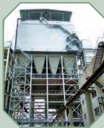
Particulate removal facilities of no. 4 unit after ultra-low emission retrofitting
