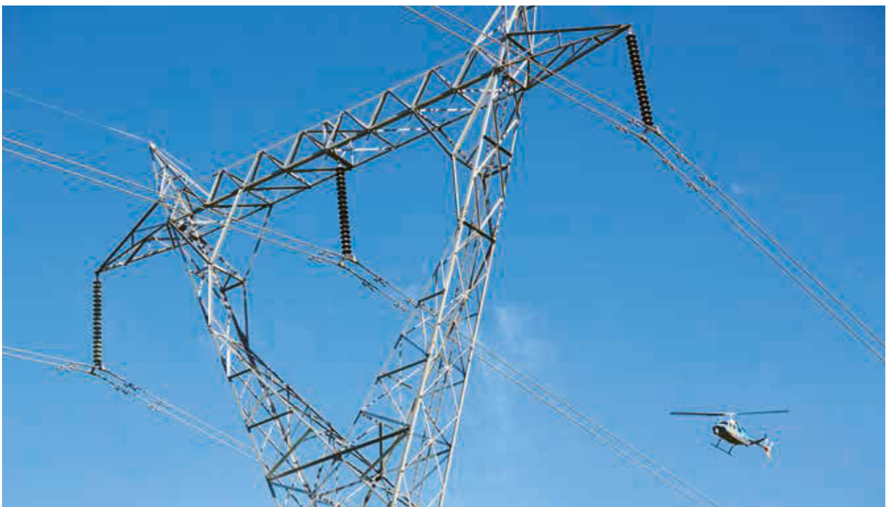
VPN uses Light Detection & Ranging technology to conduct aerial inspections to ensure network safety.
