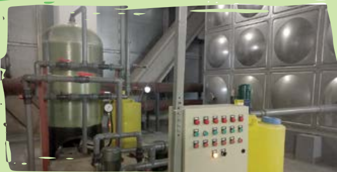
Rain water and grey water collection and reuse
