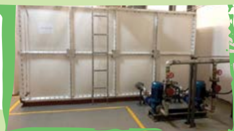
Rain water and grey water collection and reuse
