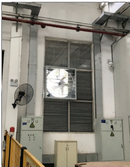
Tested the windows at the testing center and installed negative-pressure air fan and water-cooled air conditioning to improve the environment for hot work
