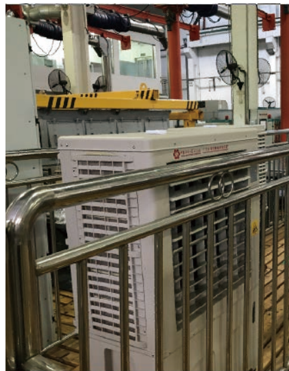
Tested the windows at the testing center and installed negative-pressure air fan and water-cooled air conditioning to improve the environment for hot work
