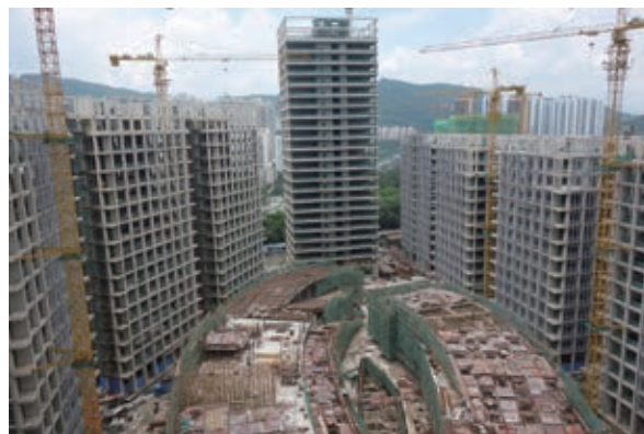
Enterprise Square – construction works in progress
