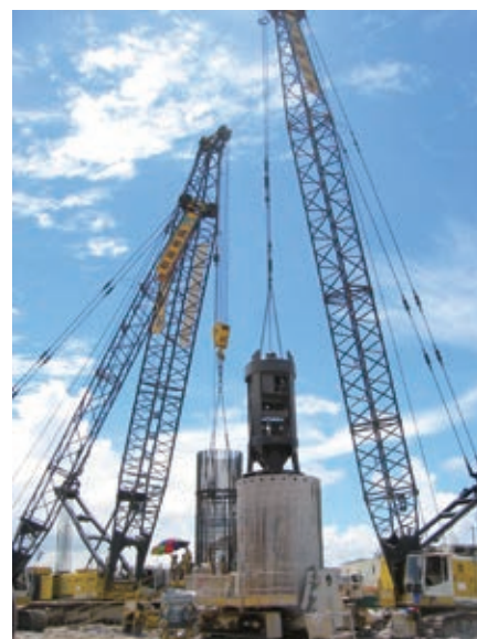
Bored piling work at a construction site undertaken by Kin Wing Foundations Limited
