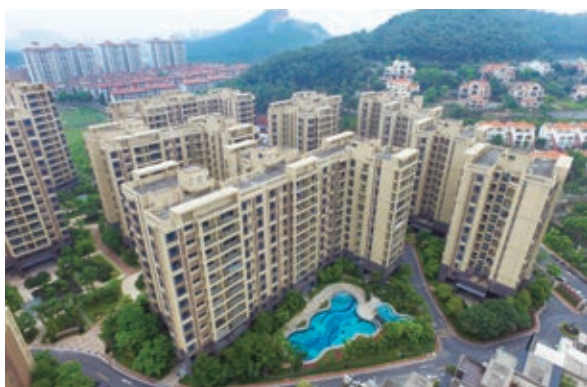
High-rise apartments under Phase 1 of Metropolitan Oasis
