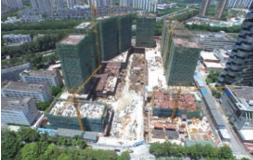
Enterprise Square – construction works in progress
