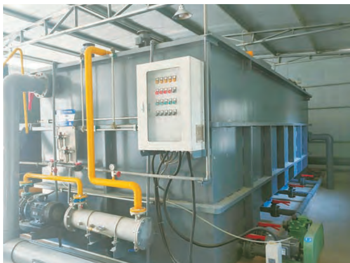
MST-EMB ultra-speed ion air flotation device for advanced wastewater treatment in Jieyang brewery
