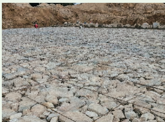
The protection slope and bank of the Jieyang project for reducing soil erosion
