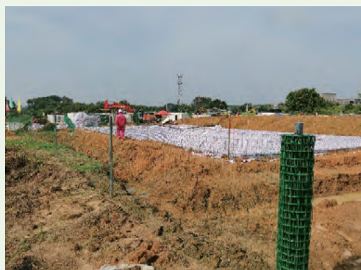
The pressure-testing water collection pool of the Jieyang project
