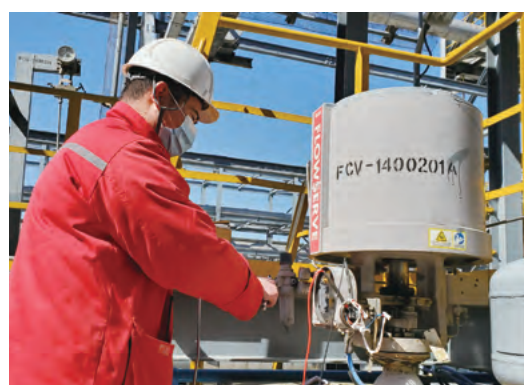
A staff of Inspection and Maintenance Center was repairing the valve positioner
