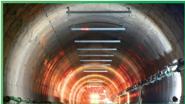
Construction of the Nation's first TBM long-range high-gradient inclined shaft of coal mine
