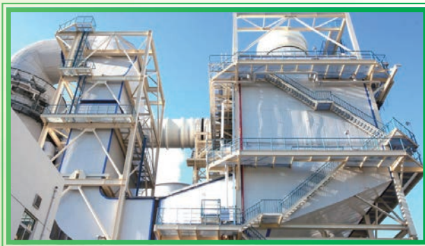
The “near-zero emission” wet dust collector equipment of Guohua Sanhe Power Plant
